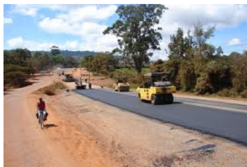
Figure 6-3. Road Construction Activity
