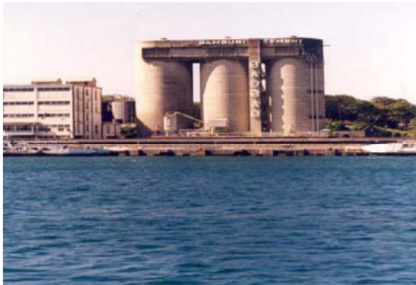
Figure 5-2.Mombasa Bulk Facilities (Cement and Flourspar)
