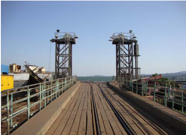
Figure 7-4. Wagon-Ferry Ramp at Port Bell
